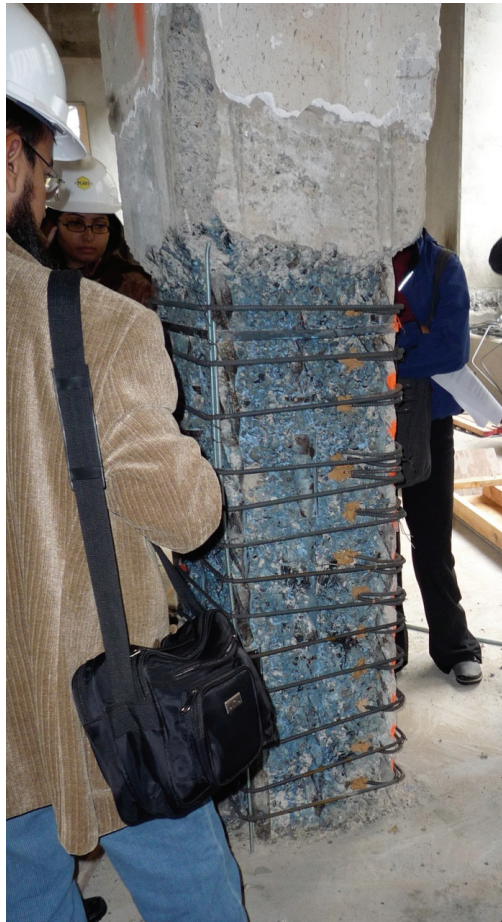
A reinforced concrete column undergoing retrofit. Photo credit: L. Thomas Tobin.
