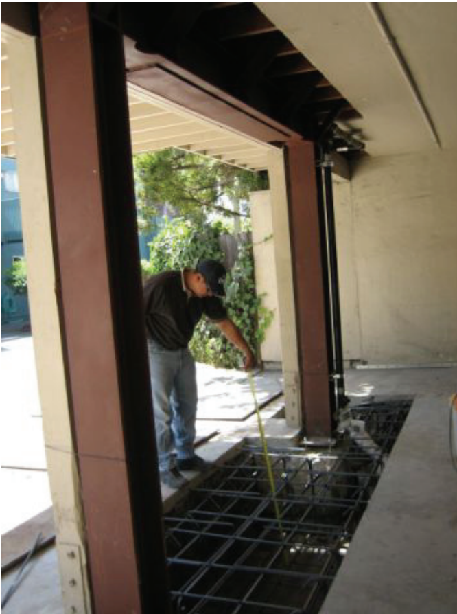
A retrofit of a soft-story residence. Photo credit: Anderson Niswander Construction.
