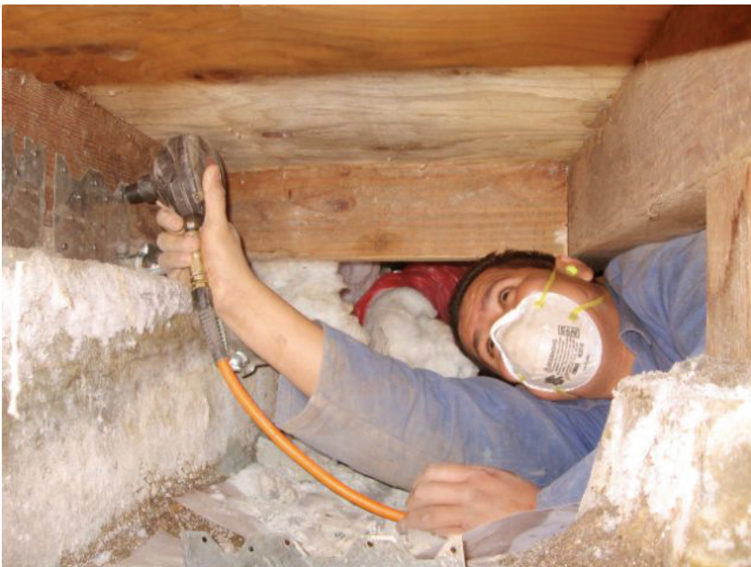
A seismic retrofit in progress. Photo credit: Anderson Niswander Construction.
