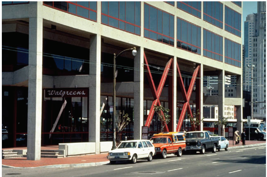
A retrofitted multi-story, soft story building. Photo credit: William Godden, Courtesy of the National Information Service for Earthquake Engineering, University of California, Berkeley.
