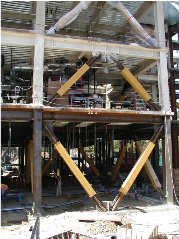
A seismic retrofit on the University of California, Berkeley, campus. Photo credit: William Godden, Courtesy of the National Information Service for Earthquake Engineering, University of California, Berkeley.
