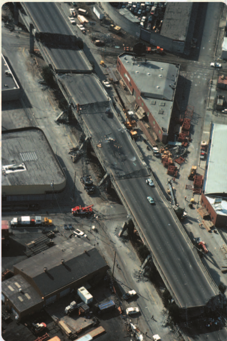
Collapsed section of the Cypress viaduct of Interstate 880 in Oakland following the magnitude 6.9 earthquake in 1989 in Loma Prieta, California.
