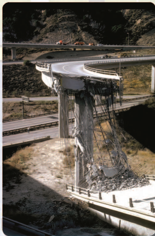
Collapse of the Interstate-5/State Highway-14 interchange showing damage north of Los Angeles caused by the 1994 magnitude 6.7 Northridge, California, earthquake. Thousands of State and County bridges were shaken at varying intensity levels during this earthquake; many required inspections.
