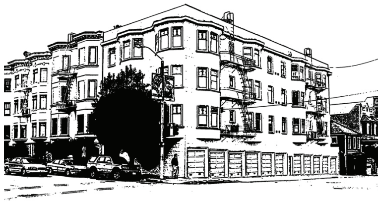
Figure 4 A typical multi-family, wood-frame soft-story building in San Francisco. Soft-story buildings can also be smaller buildings, such as single-family homes, or buildings constructed from other materials, such as concrete.
