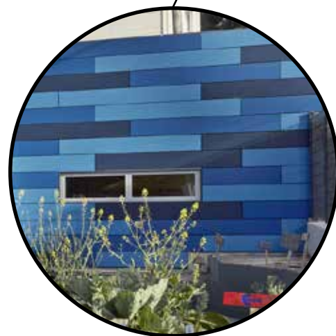
METAL PANEL CLADDING
