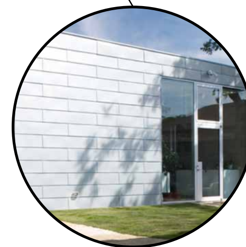
METAL PANEL CLADDING
