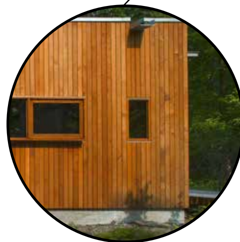
T&G WOOD WALL AND SOFFIT
