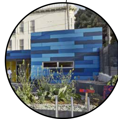
METAL PANEL CLADDING
