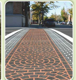
Crosswalk Treatment: Decorative crosswalks makes drivers more aware of pedestrians and provide character to the street.
