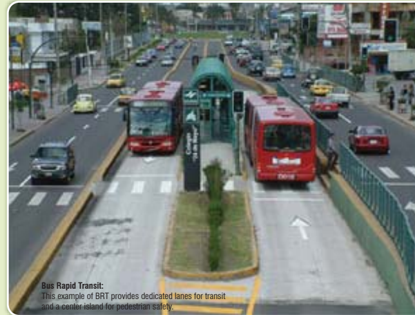
Bus Rapid Transit: This BRT design increases the pedestrian realm with landscaping.
